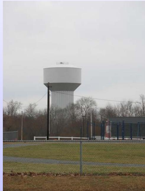
The storage tank was approximately 120-ft. to overflow, with a 40-ft. vertical sidewall height. Interior circulation piping was incorporated into the tank to avoid water stagnation and water quality degradation. Of particular interest during the siting evaluation stage for this tank was development of renderings of the visual changes the tank would have on the Design District. The project is nearing completion and expected on-line in late Spring 2009.
